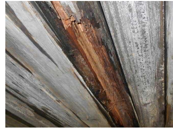
Photo 28 Interior Beam Decay
