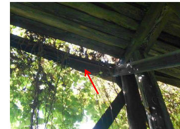
Photo 24 Failed Exterior Beam
