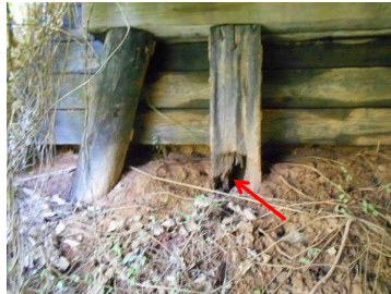
Photo 2 End Bent Pile Decay
