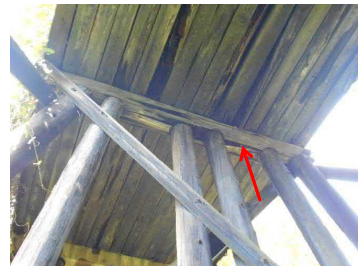
Photo 18 Split Bent Cap
