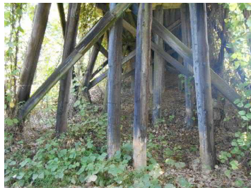
Photo 17 Typical Interior Bent
