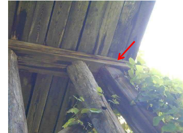
Photo 20 Split Bent Cap
