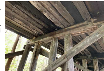
Figure 18: Interior bent cap, highlighting the splitting of the timber piles
