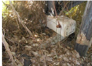
Figure 10: Timber piling resting on concrete members – a modification to the existing piles.
