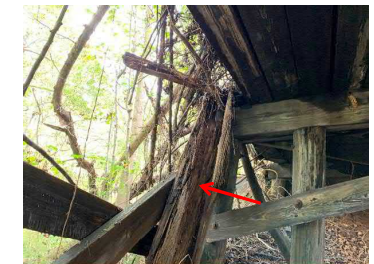
Photo 48 Completely Failed Exterior Beam
