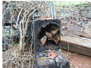
Photo 40 End Bent Backwall Decay
