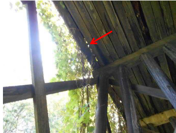
Photo 14 Rotated Exterior Beam
