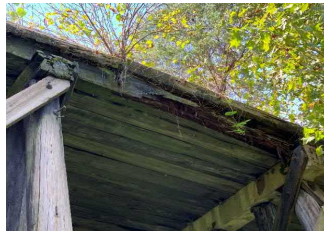
Figure 4: Significant deterioration of exterior beam, typical for exterior beams
