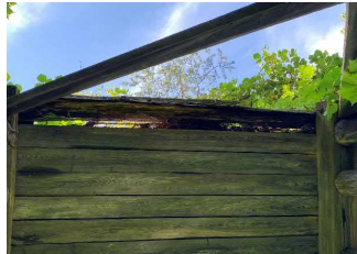
Figure 5: Exterior beam that has rotated away from the interior beams, showing visible light from above
