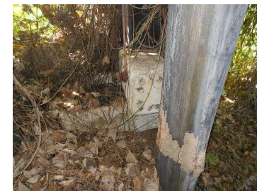
Photo 11 Bent 3 Major Pile Repair
