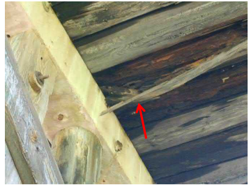
Photo 27 Damaged Interior Beam
