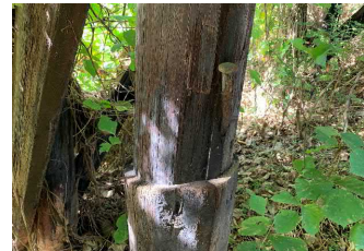
Figure 9: Timber piling that has been cut and replaced with a circular timber member and connected with a railroad tie nail.
