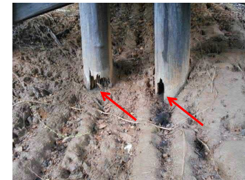
Photo 59 Section Loss in Two Timber Piles
