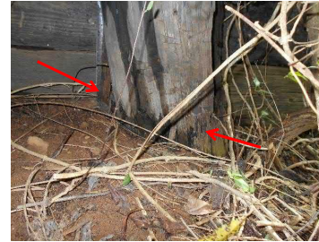
Photo 43 Damaged Timber Pile
