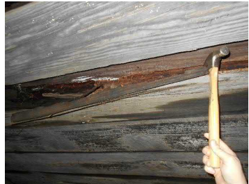
Photo 3 Interior Beam Decay
