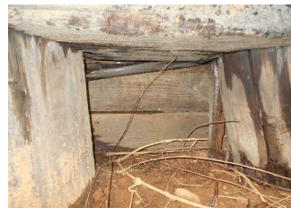
Figure 16: End Bent 1 pile cap, showing signs of decay
