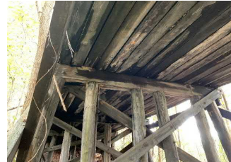
Figure 15: Interior beam showing several spans where the beams are generally in good condition
