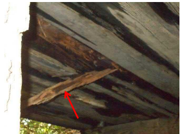
Photo 29 Damaged Interior Beam
