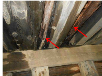
Photo 4 Interior Beam Decay
