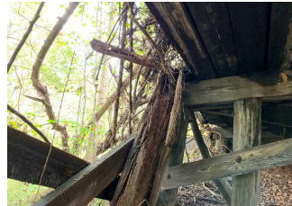
Figure 14: Complete failure in exterior beam in second span
