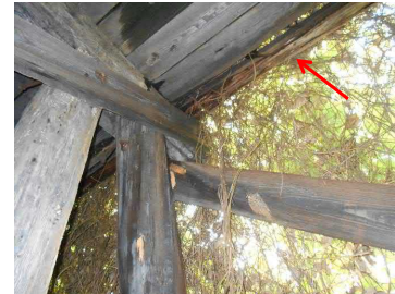
Photo 7 Failed Exterior Beam
