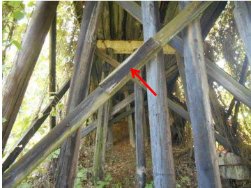
Photo 13 Spliced Cross Brace
