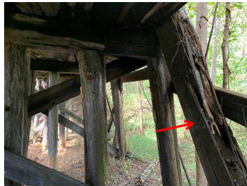
Photo 49 Completely Failed Exterior Beam
