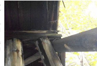
Figure 17: Interior bent cap, showing signs of deterioration at the edge
