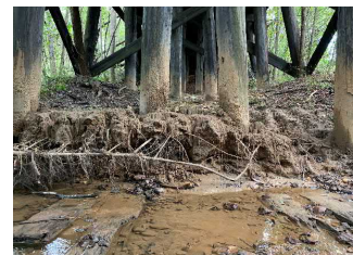
Figure 21: Stream bank scour
