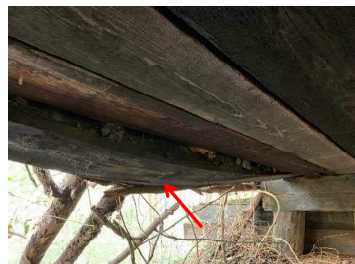
Photo 41 Failed Exterior Beam
