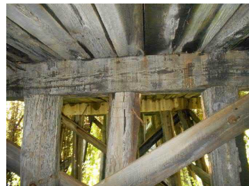
Photo 6 Typical Interior Bent
