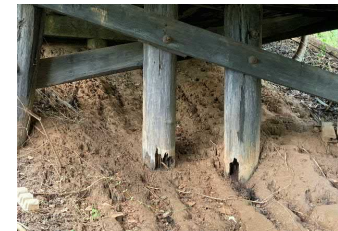
Figure 19: Significant section loss in two interior piles
