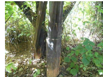
Photo 23 Typical Pile Modification
