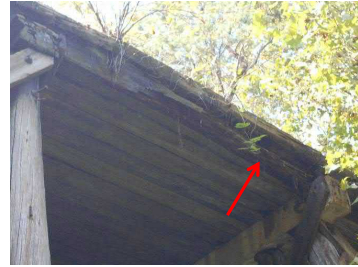
Photo 16 Failed Exterior Beam
