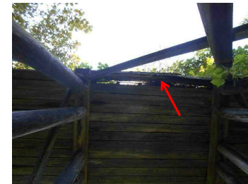
Photo 21 Failed Exterior Beam
