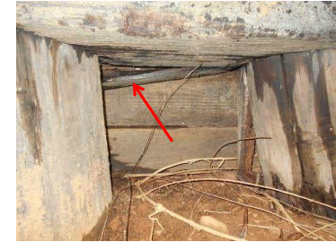
Photo 44 Damaged Timber Cap
