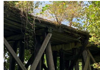
Figure 8: Timber bent cap with some section loss and decay
