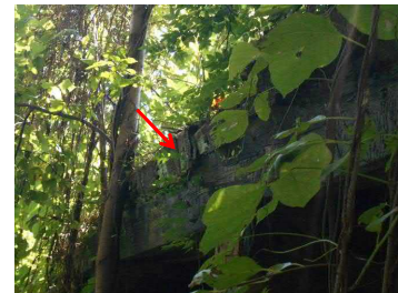
Photo 30 Rotated Exterior Beam
