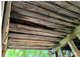
Figure 6: Interior beam showing significant section loss in span 2
