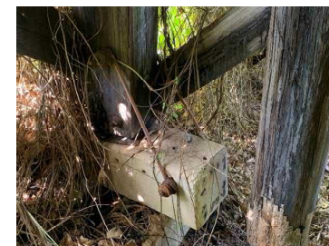
Photo 9 Bent 3 Major Pile Repair
