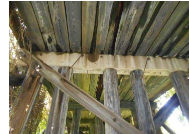
Photo 8 Concrete Bent Cap
