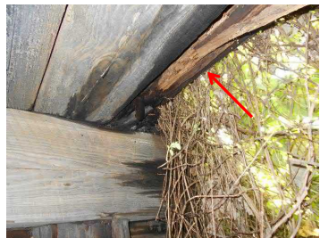
Photo 5 Decayed/Damaged Exterior Beam
