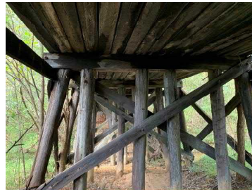
Photo 50 Typical Interior Bent
