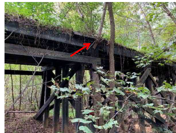
Photo 52 Tree Growing from Timber Cap
