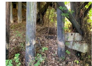
Photo 10 Bent 3 Major Pile Repair
