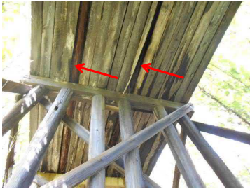
Photo 25 Damaged Interior Beams
