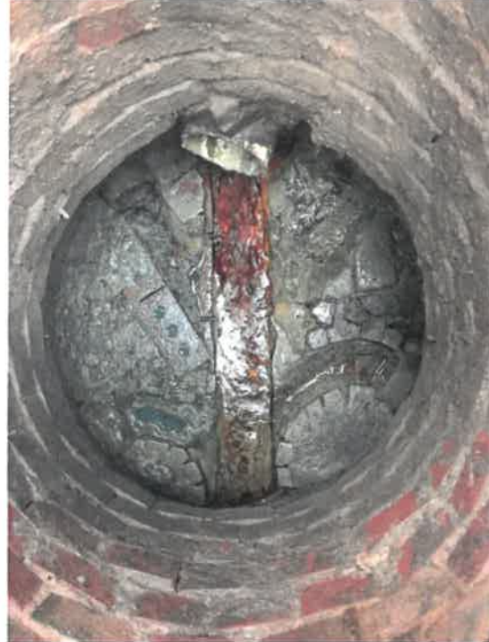
Manhole SSMH-1630 – Missing Mortar – Mud Infiltration
