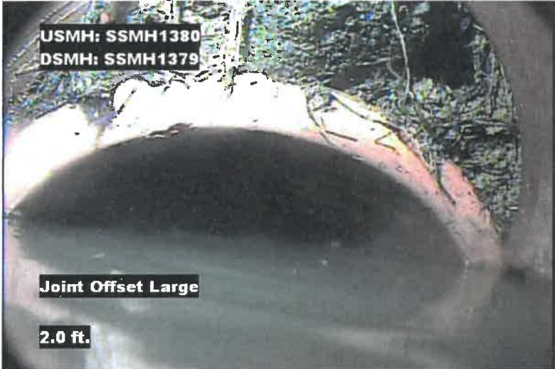
SSGM1198 – Large Offset Joint
