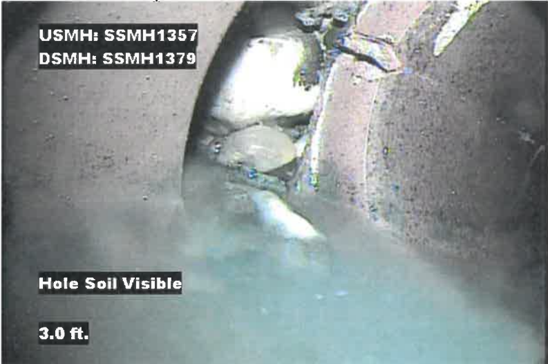
SSGM1197 – Separated Joint
