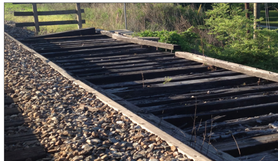
Peavine trestle bridge over NC 226
