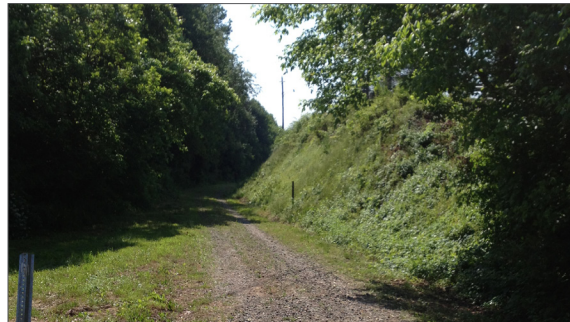
City-owned Peavine Rail Corridor
